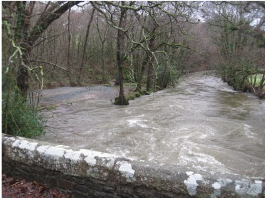
From Clapper Bridge
