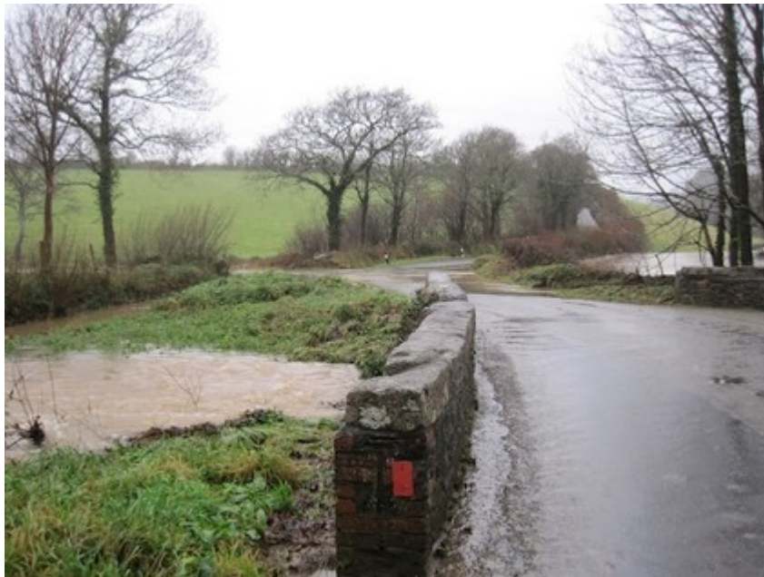
At Deans Bridge II
