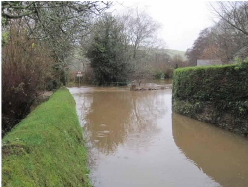
Near Pillaton Mill I
